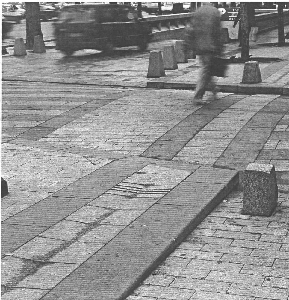
1, 2, Working drawing and detail of Métro ventilation grille. The blades are tilted to direct the air flow beyond the pedestrian way and to avoid the usual transparency of metal floorings. 3, 4, 5, Working drawing and detail views of raised kerbstone to prevent car parking along the pedestrian promenade.
