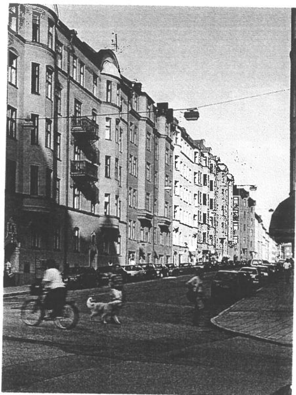
Tomtebogatan street is lined with façades in yellow-brown plaster with bulging bow windows.
