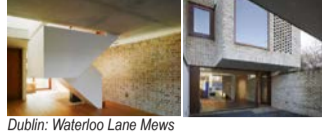
Dublin: Waterloo Lane Mews
